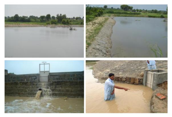
3). The existing embankments of the main reservoir were further developed with stone pitching and geo-membrane of 25000 square feet was also laid to reduce seepage. The main reservoir has been filled during the recent rains , having water storage capacity of 18 million gallon, as
