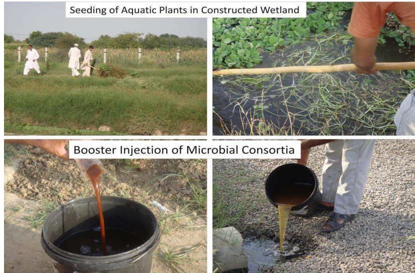
Figure 6. Application of Microbial Consortia & Seeding of Aquatic Plants in Constructed Wetland
